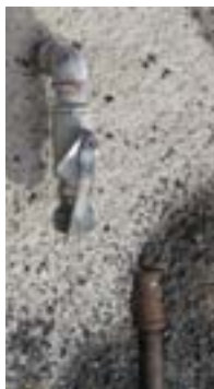
Valves such as these posed issues for employees, especially those working at night.
