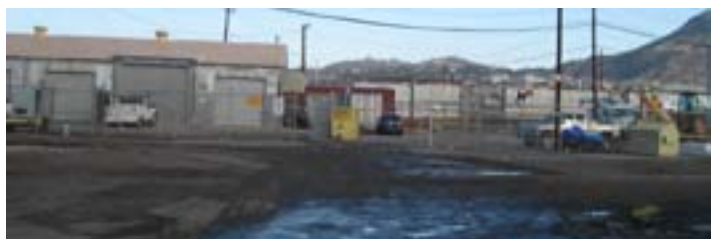
Parked cars and the absence of a stop sign posed concerns at the Langtry Street entrance to Dallas Street Yard in El Paso.
