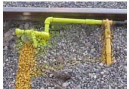
After: Valves painted fluorescent yellow
